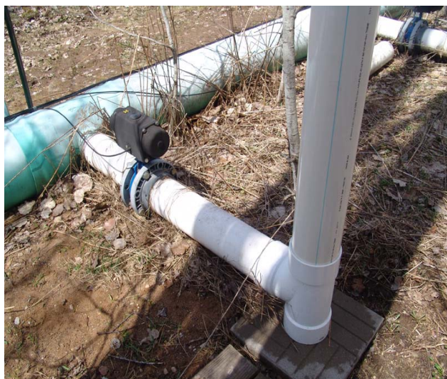
New couplings were inserted into the vertical vent pipes and these were placed on a cement pad to support the taller VVPs.
